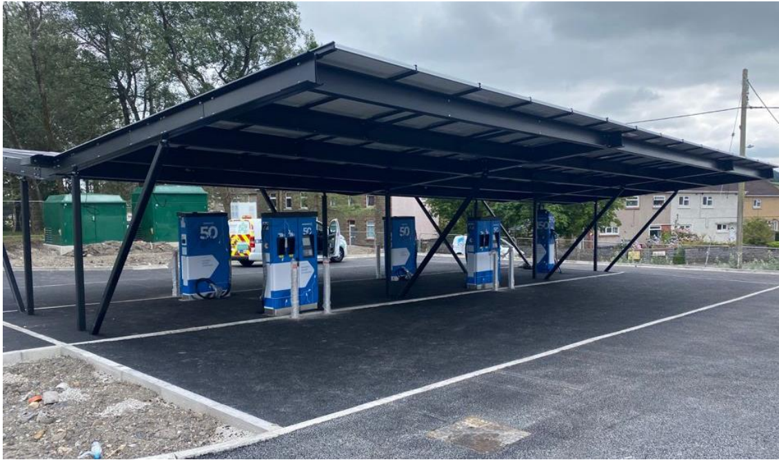
Figure 16 - Cross Hands EV Charging Hub (in construction)
