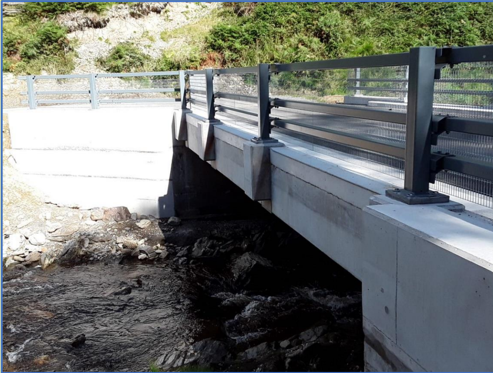
Doethie bridge replacement 2021
